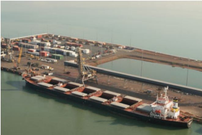
Stockpiled iron ore is loaded from the East Arm Wharf's new $24 million bulk handling facility.
