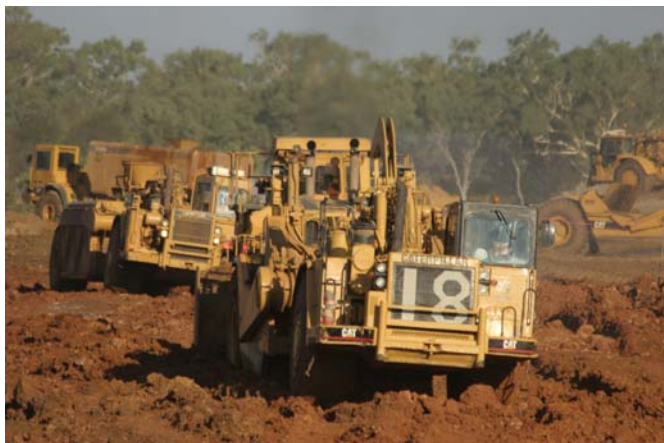
Heavy machinery at work on the McArthur River mine site.
