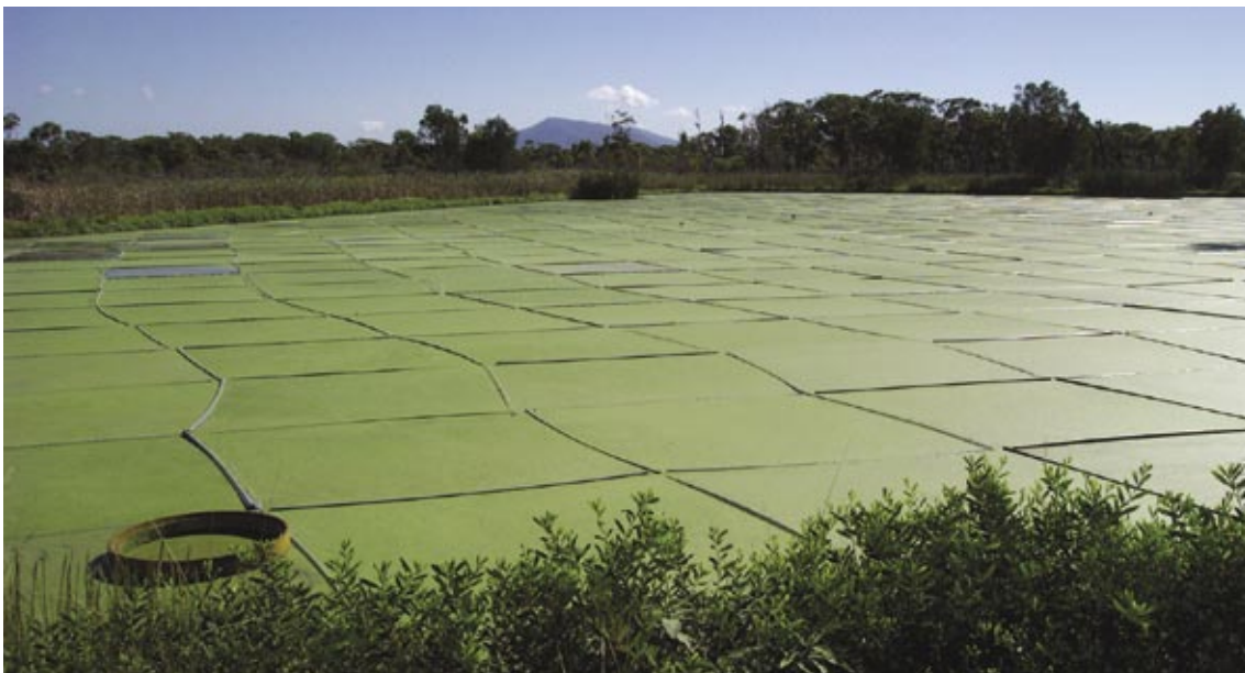
Photo 1. Harrington Sewerage Treatment Works, NSW: 0.7 ha DWT lagoon showing floating grid network for containing duckweed.
